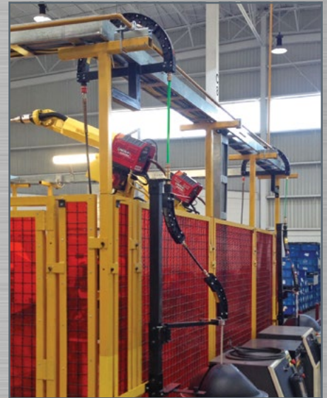
180° Modules installed on cell with two robots and the Non-Stop™ Wire Dispensing System
